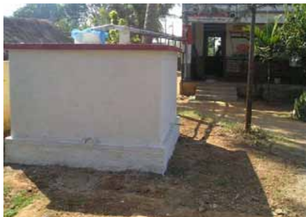
Rainwater storage tank
