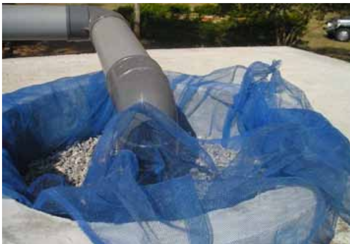
A good filter with mesh and gravel on top
